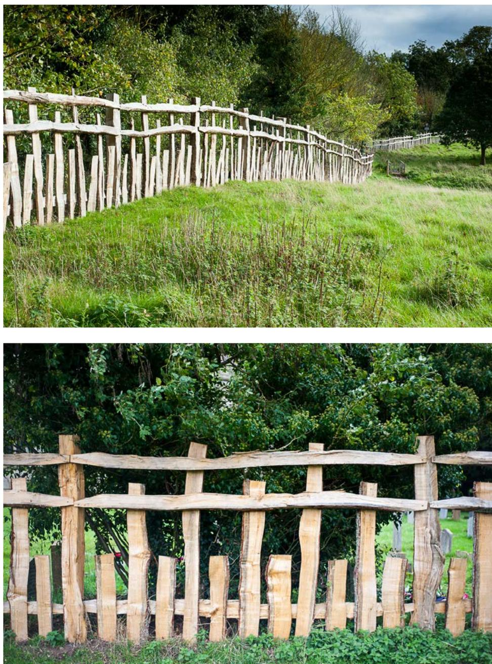
Figure 5: New deer-park fencing made by cleaving oak at Charlecote Park in Warwickshire showing pales of three heights supported by three rails. The tallest posts are 6 ft. (1.83 m) high. The fence is not set on a bank and ditch system. Photographs by the author.
