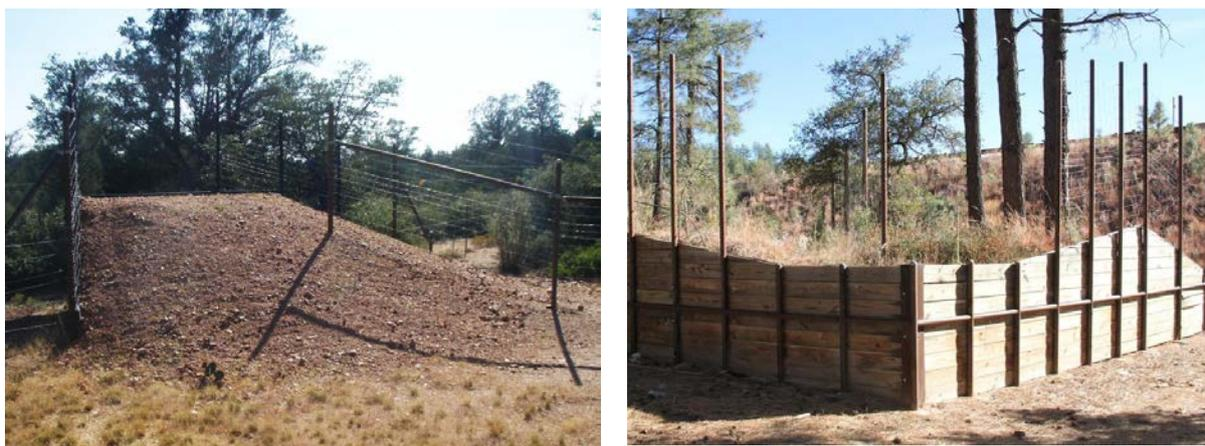
Figure 14: ‘Jump-outs’ in the US designed to enable large mammals such as deer/elk trapped on the highway to escape and not return: (left) a ramp on the highway side up to a drop; (right) a wooden revetment with wire supported by poles directing trapped animals from the highway at the top, to the one-way drop, and thereafter to cross the highway via an underpass. Photographs courtesy of the Arizona Game and Fish Department.
